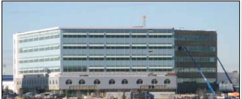
45,000 SQ FT X 6 Floors + Underground No-vented with CO monitoring (7 heaters)
