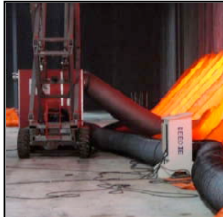
TRENCH 200' X 10'W X 6'D 3' of Frost in 4 days
